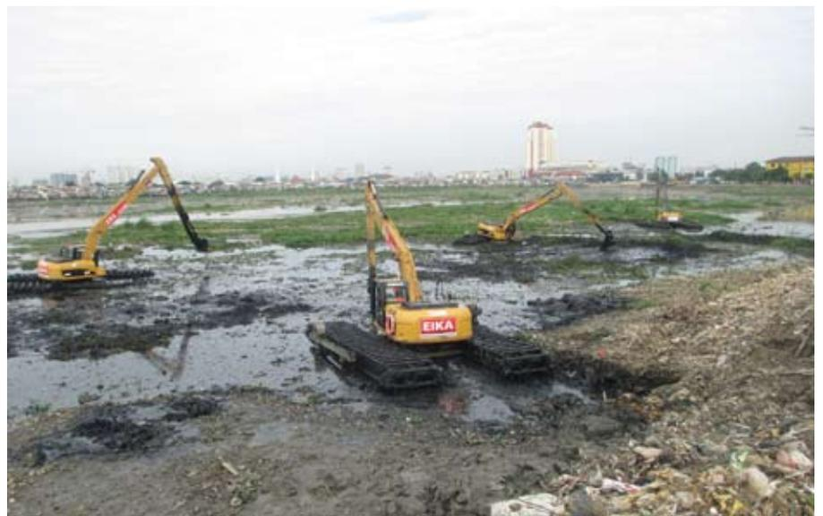
reservoirs unable to store the excess water, and the canals could not drain it properly either. EIK's amphibious undercarriage design features the multi-synchronous drive system, which provides excellent tracking ability in soft and high viscosity terrain; coupled with the pontoon's low ground pressure, the amphibious excavators excelled and thrive in this challenging environment.
