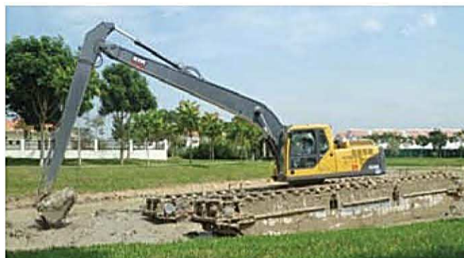
A Volvo EC210 excavator in amphibious long boom-and-arm dredging guise.
